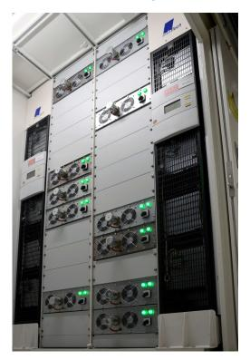
A segment of the IT-Area of the MDC40 with load resistances. Full power consumption is sumulated through 20 load resistances per 3KW.
